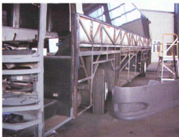
Panel removal from Bus using BTB Tool & "V-S" blades
